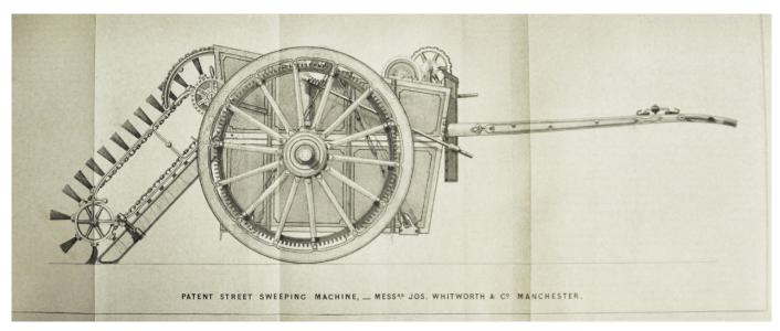
Fig. 2 Whitworth's patent street sweeping machine
