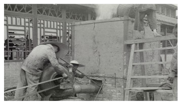
Fig. 1 Men at work at a cupola furnace in the Central Machine Works in Chengdu, SW China, May 1943 (Photograph: Joseph Needham).
