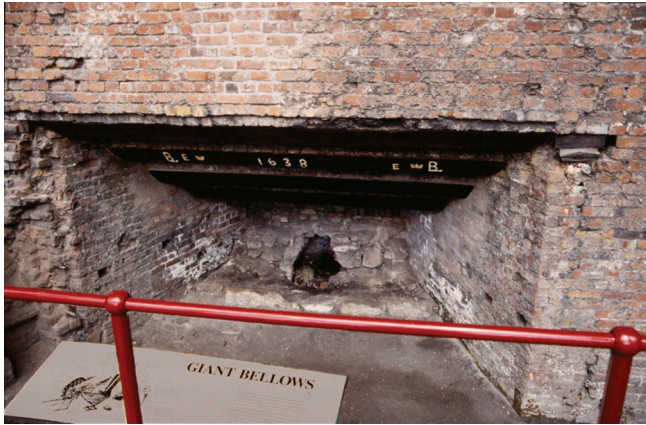
Figure 84: The bellows arch of Abraham Darby's furnace at Coalbrookdale, Shropshire.
