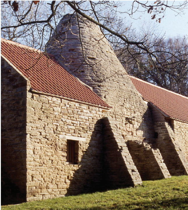
Figure 86: The early-18th-century cementation furnace at Derwentcote, Co Durham, with attached working buildings.
